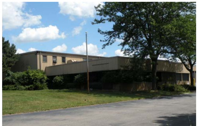
Haggerty Road has a number of underutilized parcels that would be ideal for redevelopment along this mixed-use corridor
