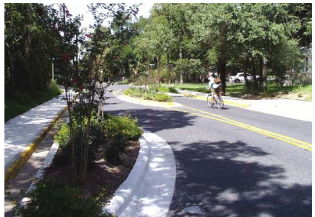
Examples of traffic calming: a speed hump, choker and chicane (from top to bottom)
