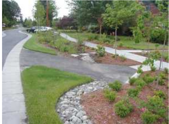
Low Impact Development techniques can help a site manage its storm water on site
