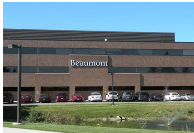
Successful businesses and employment centers are critical for the economic future of West Bloomfield
