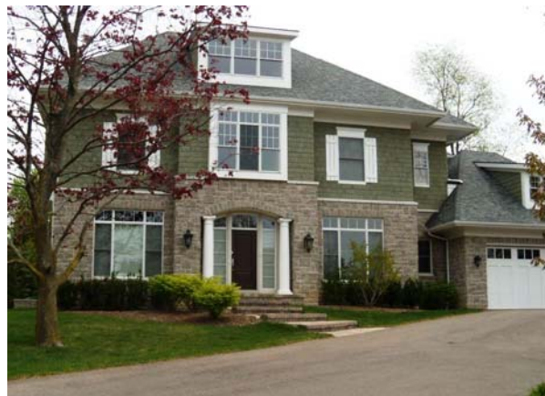
Infill residential development should respect the character of neighborhoods
