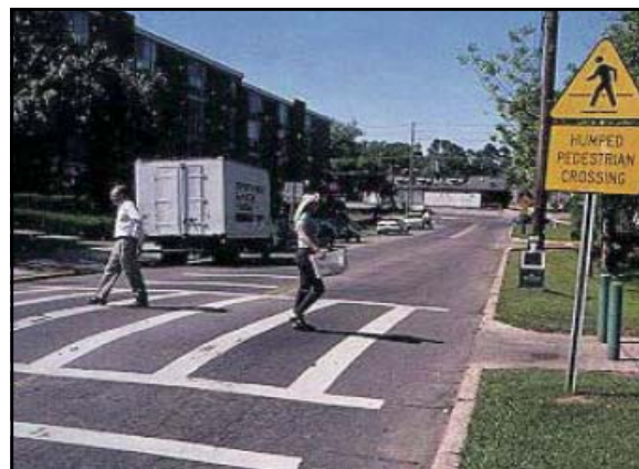
Examples of design elements to improve pedestrian safety including bump outs, raised crosswalks, and signage
