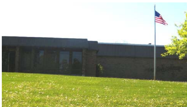
The Water and Sewer Department is located off of Haggerty Road
