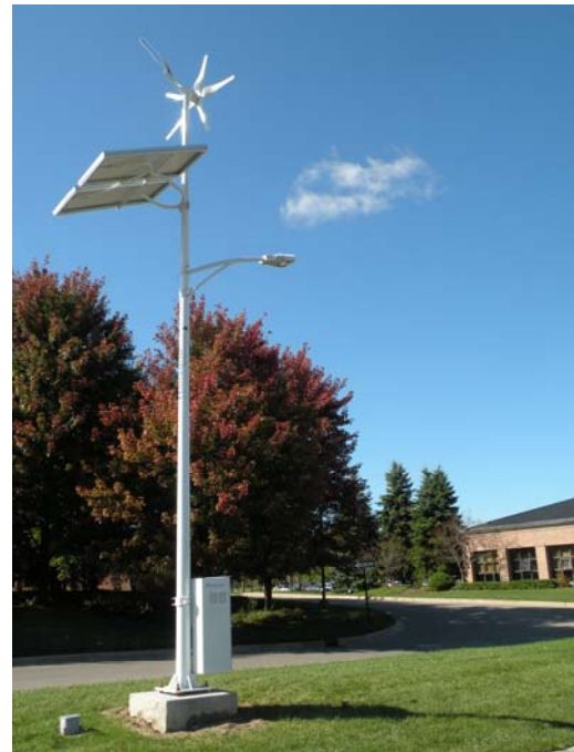
West Bloomfield Township Hall is home to the nation's first wind/solar lighting system
