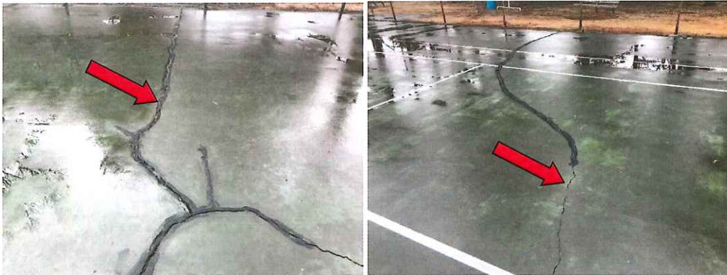
Figure 9: Images of new pavement cracking continuing past limits of previous emulsified asphalt repairs. Existing repairs have failed.
