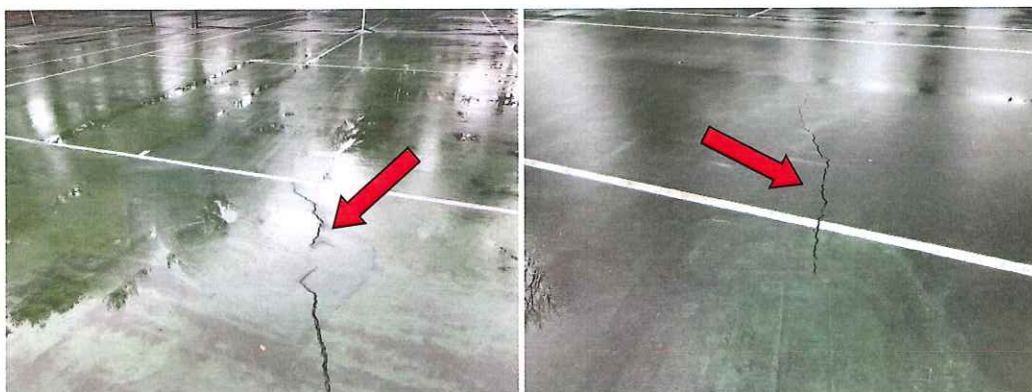
Figure 8: Images of new pavement cracking continuing past limits of previous membrane repair system. Membrane repairs have started to fail.
