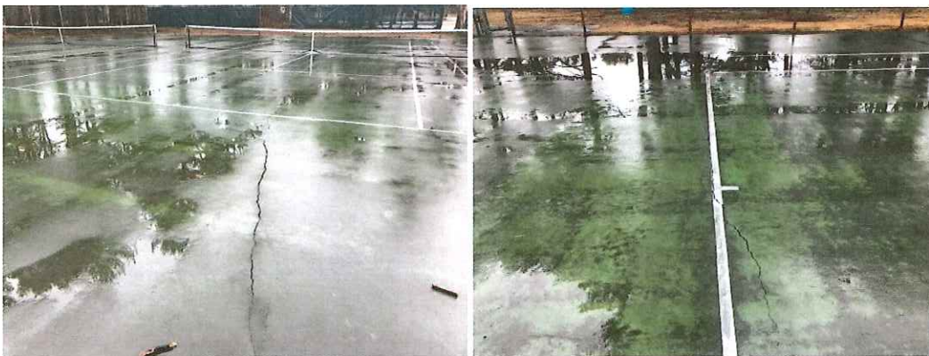
Figure 10: Images of court acrylic surface fading and staining.
