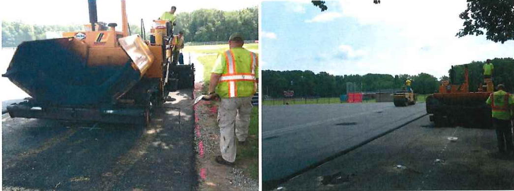
Figure 12: Images of new pavement overlay.
