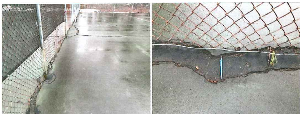
Figure 6: Images of pavement radial cracking along fence line (crack widths of over 4").
