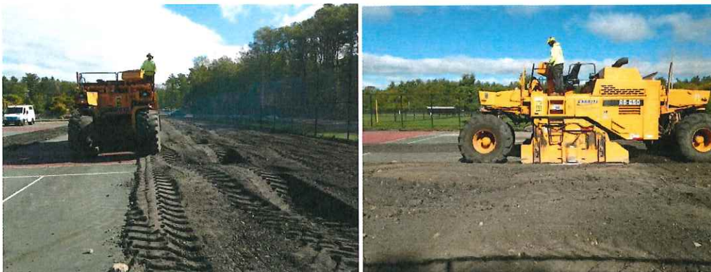
Figure 13: Images of full depth pavement reconstruction.
