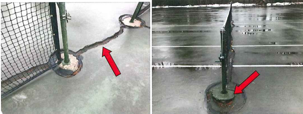
Figure 7: Images of pavement radial cracking along net line (crack widths of 2" - 4"). Emulsified asphalt crack repairs have failed, and water intrusion resulted in post foundation heaves.
