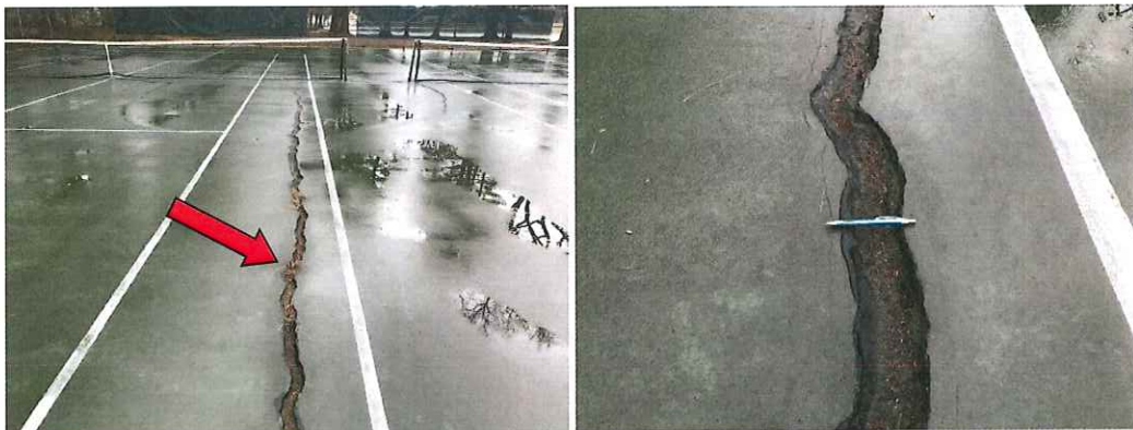
Figure 5: Images of pavement structural cracking along cold joint (crack widths 2" – 4").
