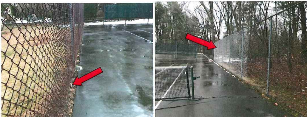
Figure 2: Images of existing fencing showing no bottom railing and sections with repaired fabric.
