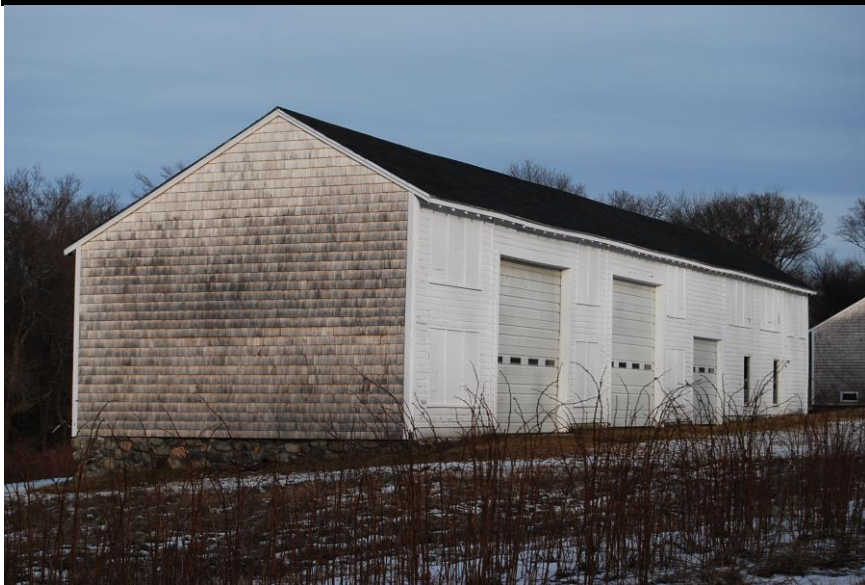
Photo 3. Iori west barn. View facing east. (WNH.176)
