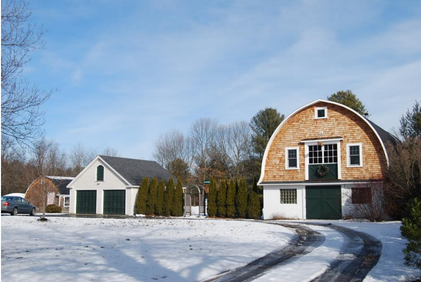
VIEW FACING NORTHEAST. LEFT TO RIGHT: SHED; GARAGE; BARN
