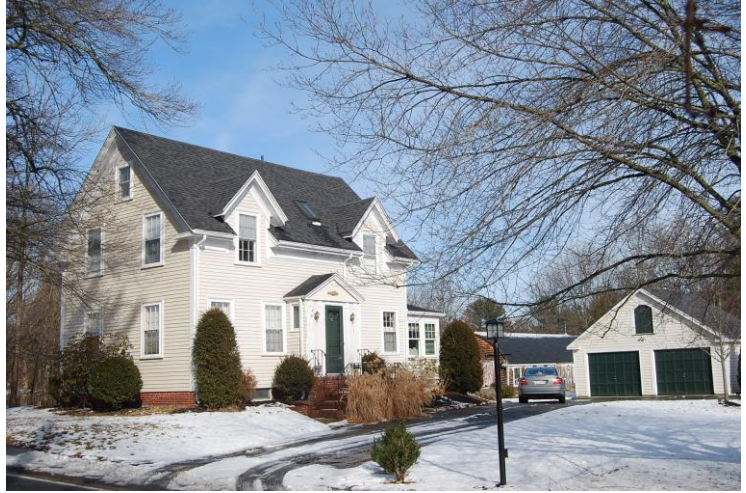
West and façade (south) elevation.
