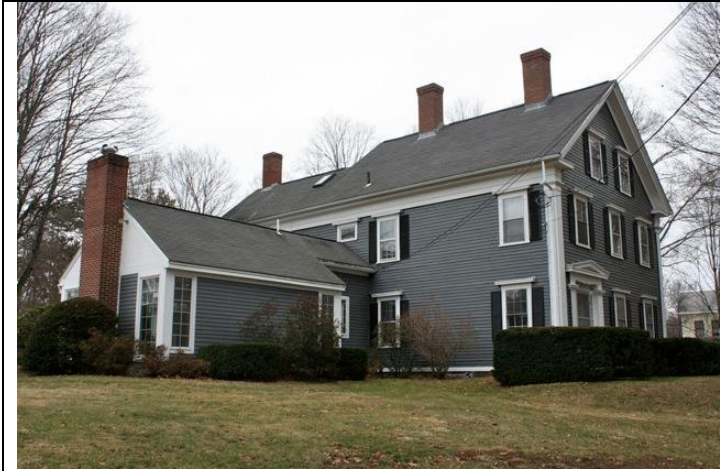
Photo 2. East and façade (north) elevations.
