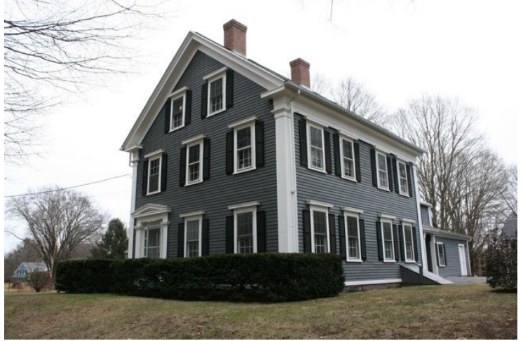
Façade (north) and west elevations.
