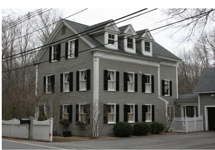
Façade (west) and south elevations.
