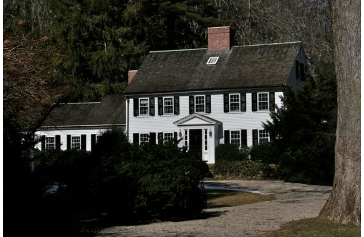
Photo 1. Façade (south) elevation.
