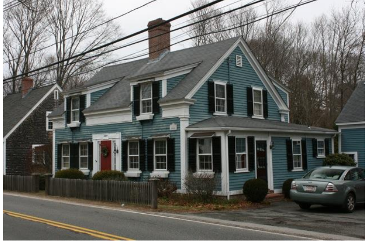
Façade (west) and south elevations.
