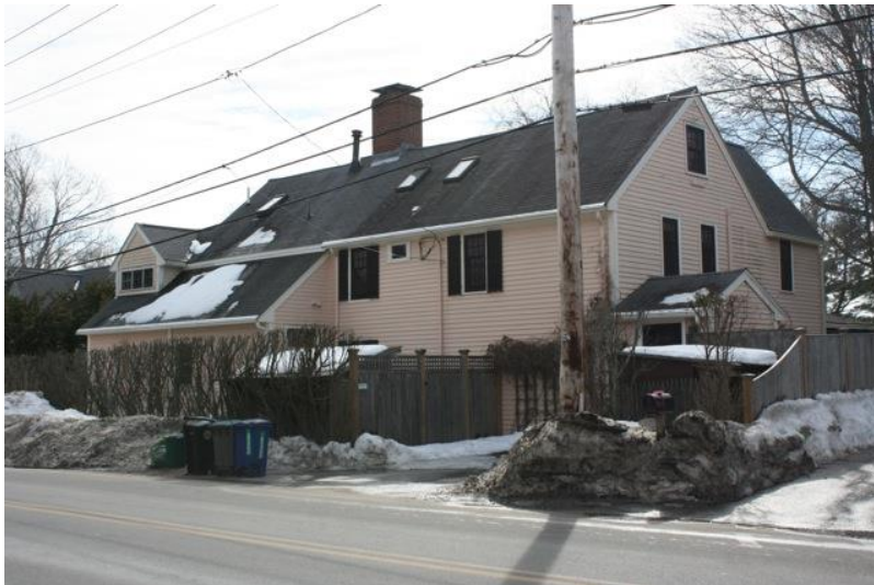
Photo 2. Rear (north) and west elevations.
