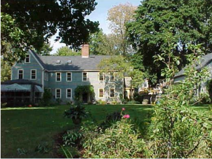
Photo 3. South elevation. Assessor's Record.
