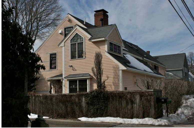
Rear (north) and east elevations.
