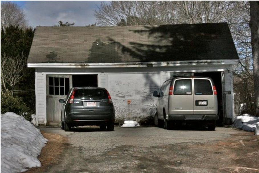
Garage. Façade (south) elevation.
