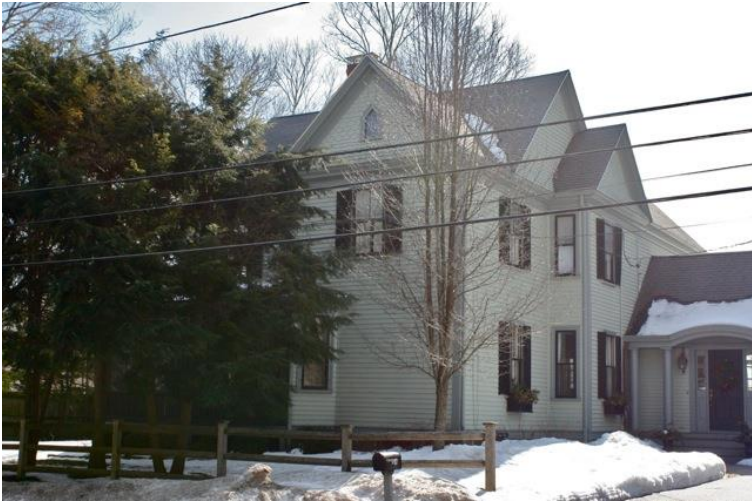
Photo 2. Façade (north) and west elevations
