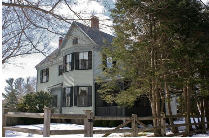
East and façade (north) elevations.
