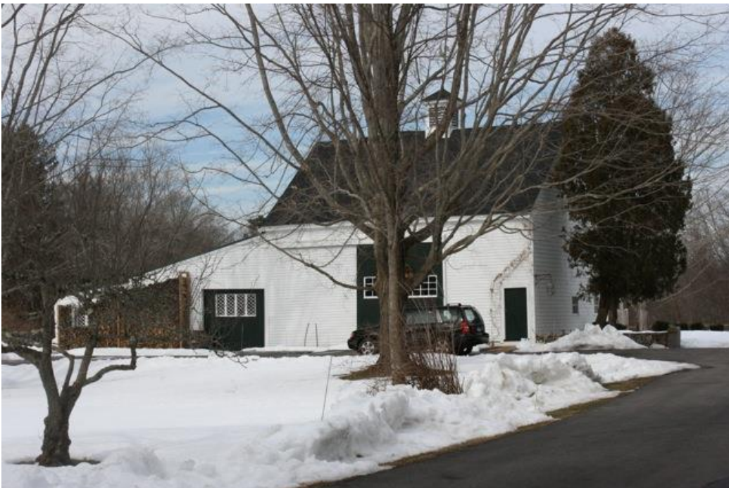
Barn, south elevation.
