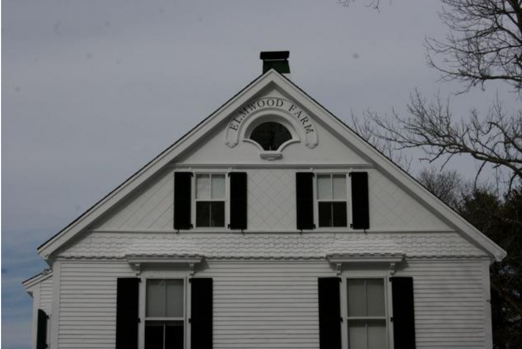
Façade (south) elevation. Detail.
