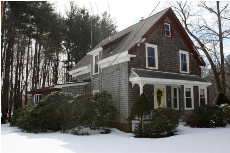
North and façade (west) elevations.
