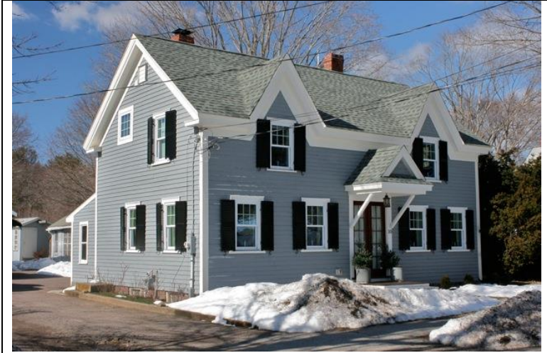
Façade (east) and south elevations.
