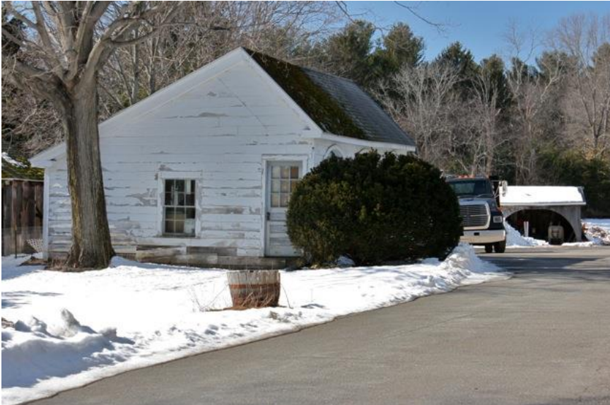
Garage. East and north (main) elevations.
