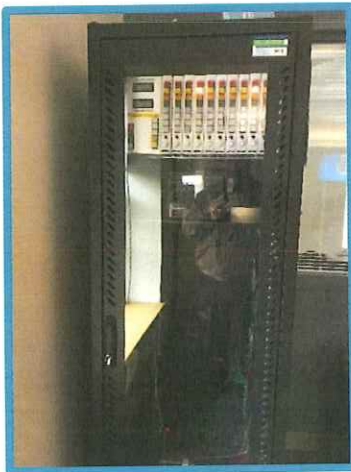
Figure 6 Keltron Fire Alarm Annunciator
