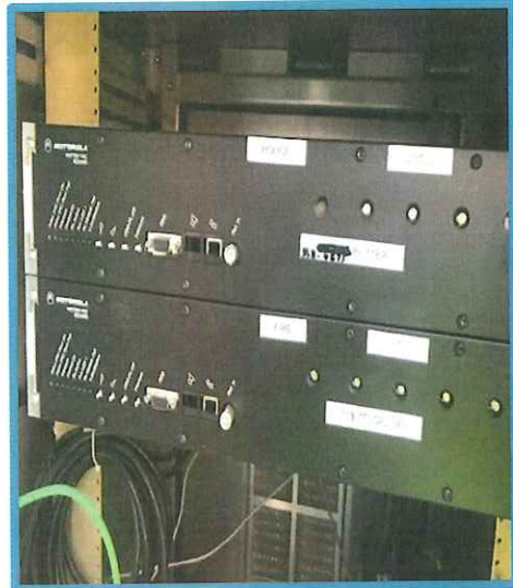
Figure 38 Burnham Road Astro Tac Receivers
