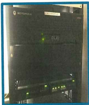
Figure 34 UHF MTR 3000 & Duplexer
