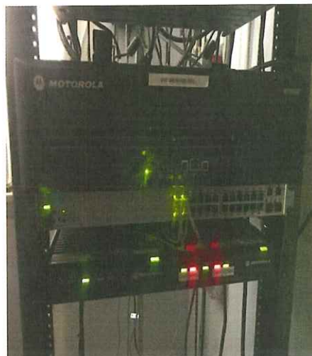
Figure 37 VHF MTR 3000 and Multi-Switch & Voting Equipment
