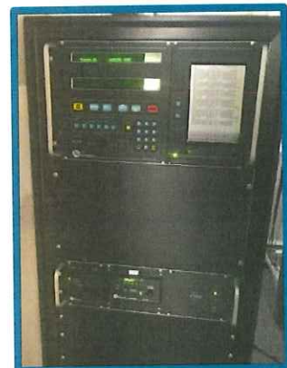
Figure 33 Vision 21 Fire Alarm Receiver
