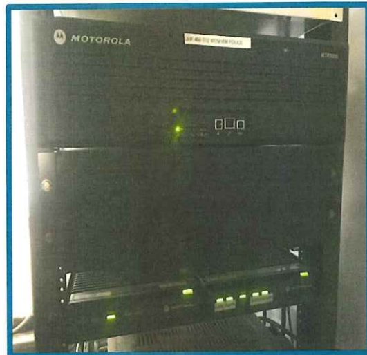
Figure 36 UHF MTR 3000 & Duplexer PD
