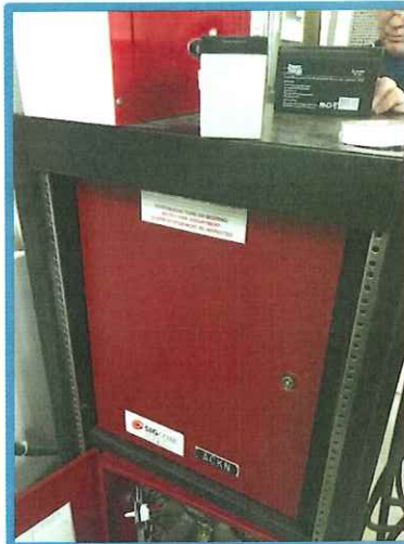
Figure 41 Sig Com Fire Alarm Box
