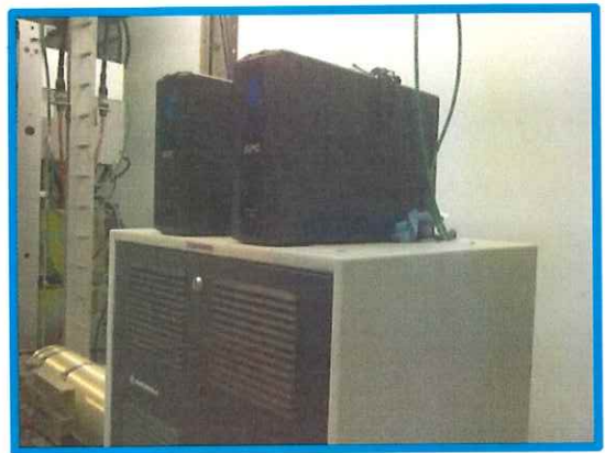
Figure 11 UPS Back Up Danvers Hospital Site
