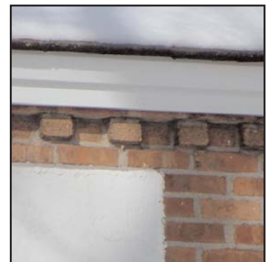
Dentil brick work
