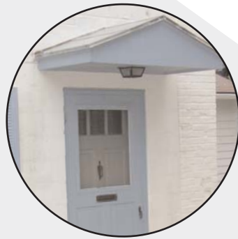
Cantilevered overhang
