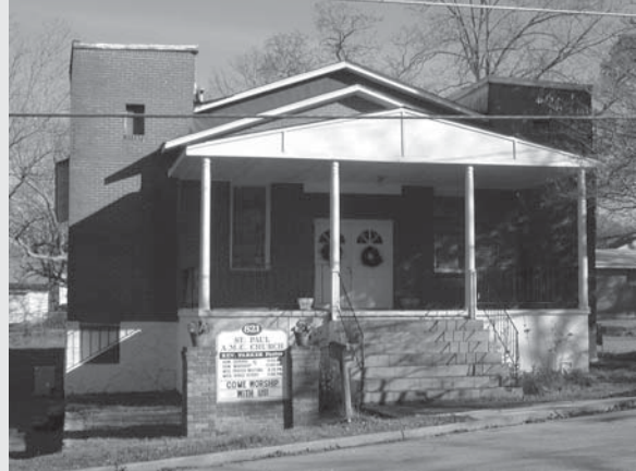
The St. Paul A.M.E. Church in Shermantown was built circa 1950 and features a central, gabled main room with bell towers flanking the front facade.
