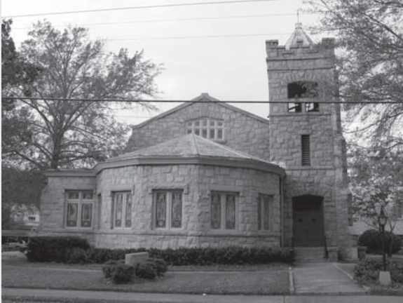
The Stone Mountain United Methodist Church, constructed in 1909, is an impressive ashlar granite building.
