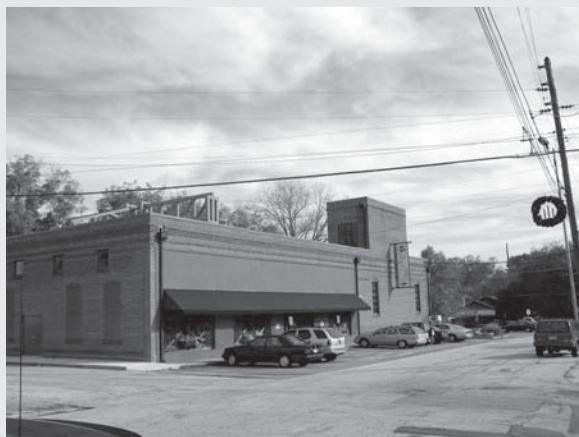
The circa 1920 A.R.T. Station was originally the trolley station for Stone Mountain.
