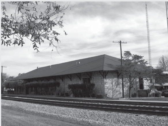
The Stone Mountain City Hall, originally the Georgia Railroad Depot, was built in two phases of construction (circa 1870s & 1914).
