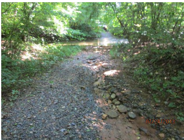
Photograph 41: View of ford crossing on site 19 on Ostin Creek. Channelized flow through crossing is a potential source of sediment.
