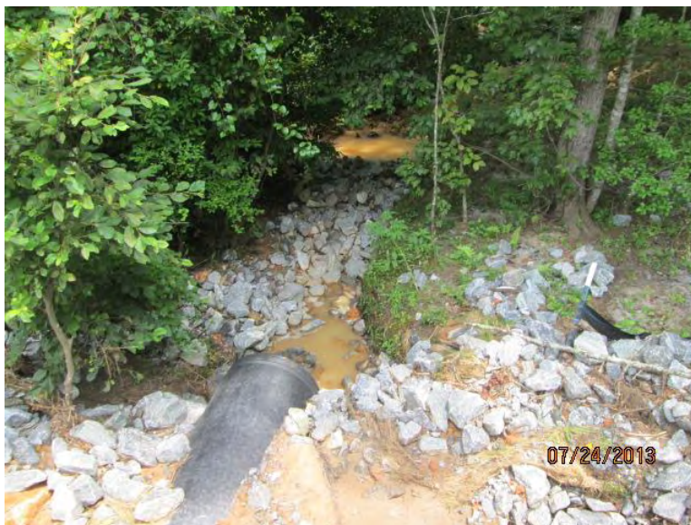
Photograph 60: View of discharge from pond at Site 22. The banks appear to be eroding, and the rip-rap also appears to be unstable.
