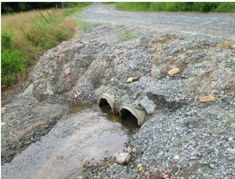
Photograph 67: View of culverts at site 26 leading to the Rash Creek. A third culvert is buried beneath the gravel.
