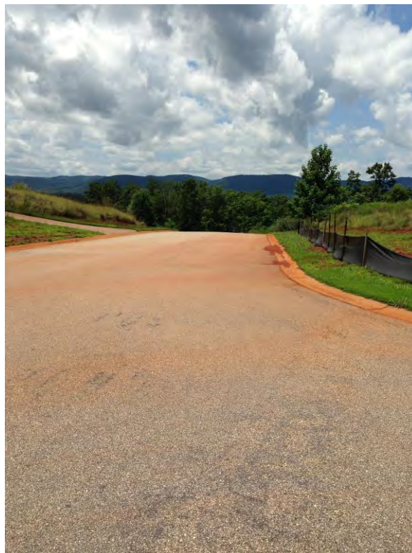
Photograph 92: View of street within Lake Adger Development following a rainfall event. Note the red sediment stained pavement indicative of sediment laden runoff.
