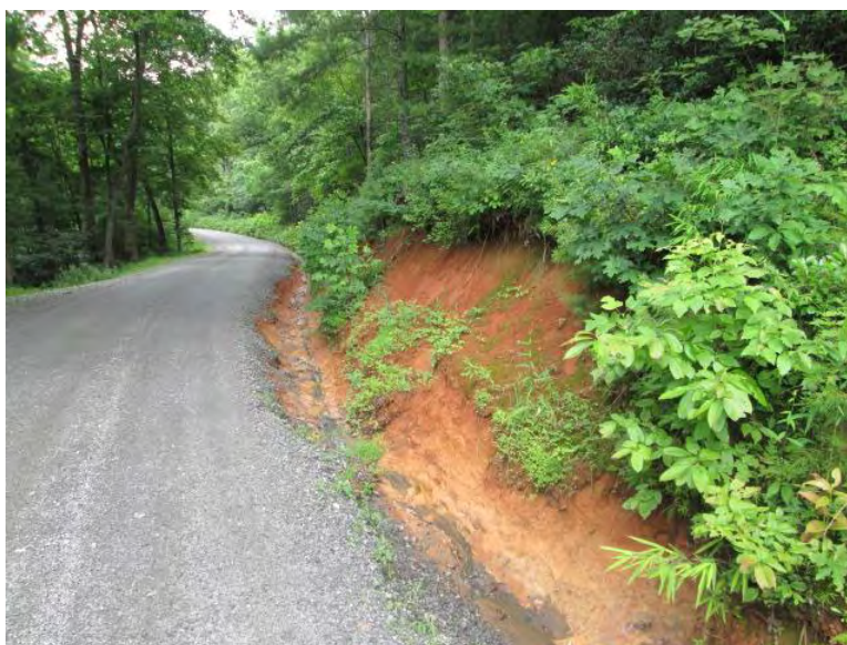
Photograph 63: Representative view of eroding ditch along Raegan Jackson Road near Panther Creek Site 6.
