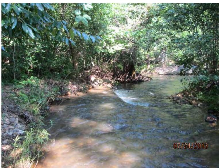
Photograph 47: Typical view of restored reach of Ostin Creek on Site 15. Log vane installed on leftbank to divert flow off leftbank.
