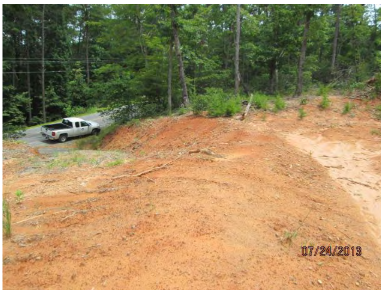
Photograph 61: View of upland area near Site 22. The exposed soil is likely contributing sediment to the pond and Ostin Creek
