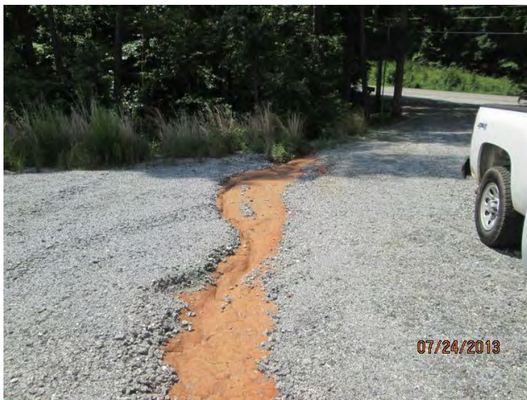
Photograph 74: Representative view of erosion on gravel road near power station near the intersection of Sylvan Lane and Silver Creek Road. Runoff from this area drains to Silver Creek.
