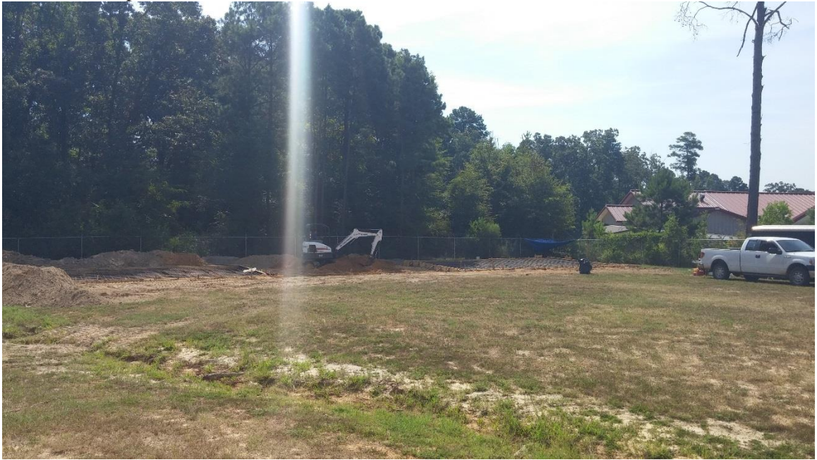
Arkansas road plant Construction
