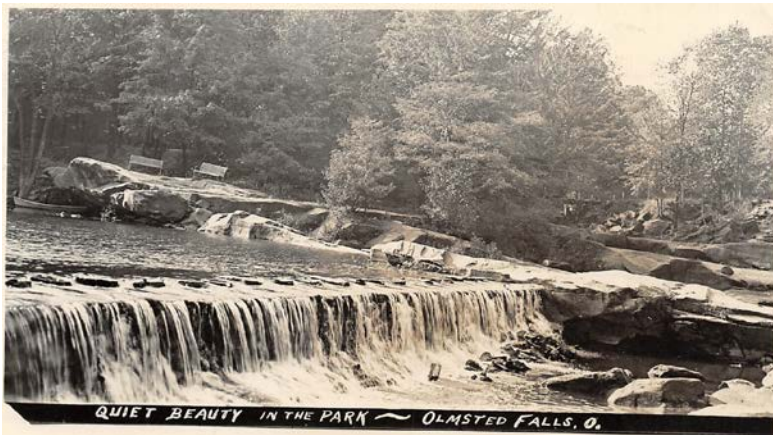
This mid-1950s postcard, called “Quiet Beauty in the Park,” shows the dam built along Rocky River in 1930 to form a swimming hole and ice skating rink. Note the stepping stones on top to allow people to walk from one side of the river to the other when the water level was not high.
