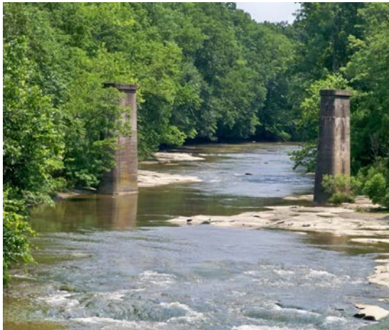
These pillars were built for a bridge to carry trains over Rocky River for a railroad that was never built.
