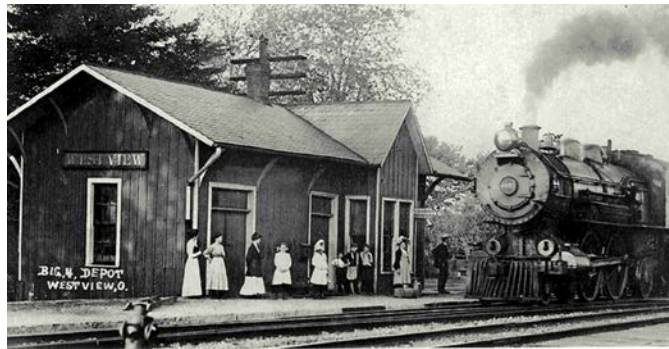
This photo shows a train arriving at the West View depot of what then was the Big Four Railroad in the late 1800s.
