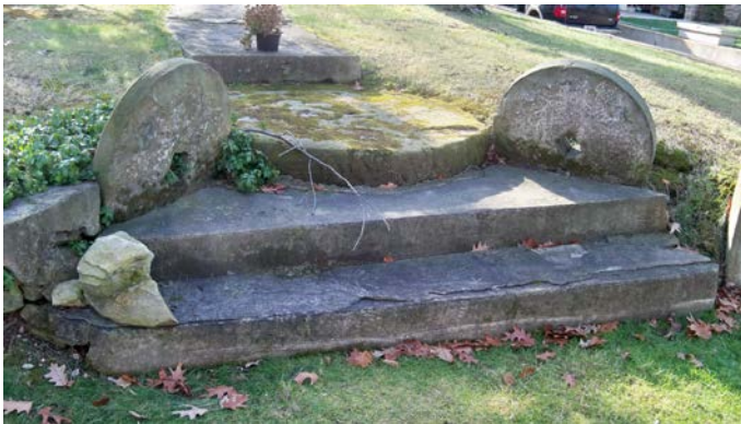
This set of steps at a residence near the former West View quarry makes use of three grindstones and long sandstone blocks evidently from the quarry.
