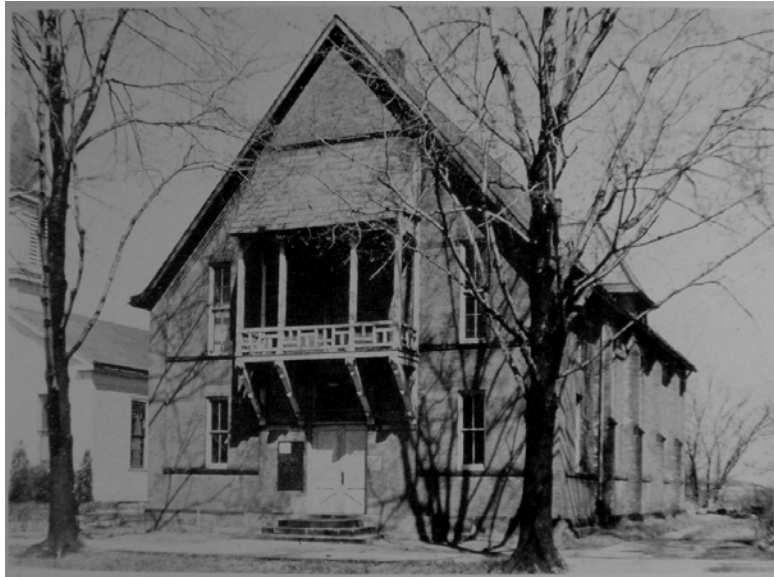
The Town Hall stood next to the Congregational Church (to the left) from 1883 until 1939. The site now is occupied by the Moosehead restaurant.
