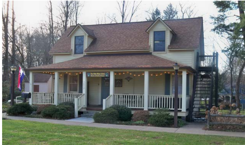
August Von Brause lived in this house and worked as a blacksmith in his shop next door. The building at 7932 Main Street in Olmsted Falls housed the Jenkins Senior Center for many years. It now is home to the Olde Wine Cellar.
