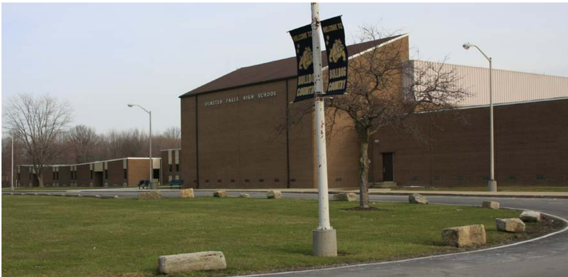
Before recent construction began to expand the high school, this is how it looked with the auditorium in the foreground.
