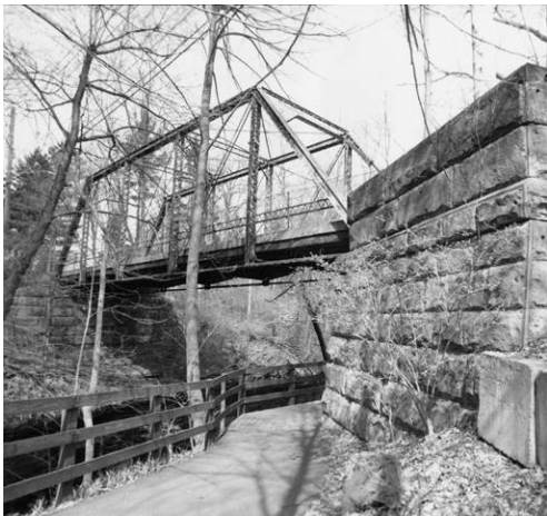
This photo of the bridge from 1997 shows the walking trail underneath.
