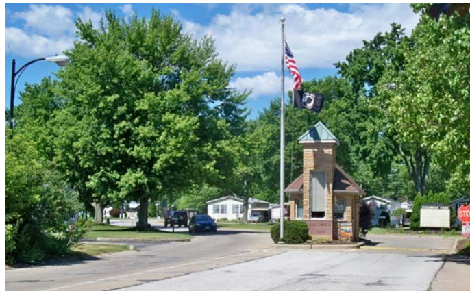
Drivers entering Columbia Park must pass this security checkpoint.
