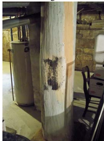
This "old tree trunk" supports a main beam.
