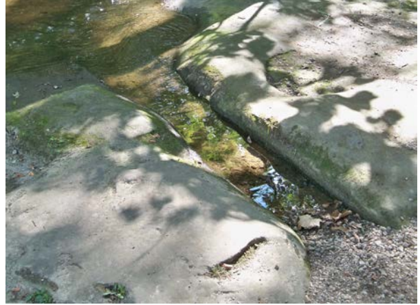
The photo on the left shows a diagonal groove on the side of Inscription Rock that might have helped Lemuel Hoadley and John Barnum secure planks for the dam for their mill on Plum Creek. On the right is part of the hand-chiseled sluice carved into the rock on the opposite side of the creek.
