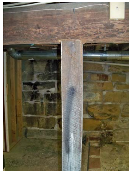
Above right, thick wooden beams are in the basement. Left, quarried sandstone and fieldstone both form parts of the basement walls.
