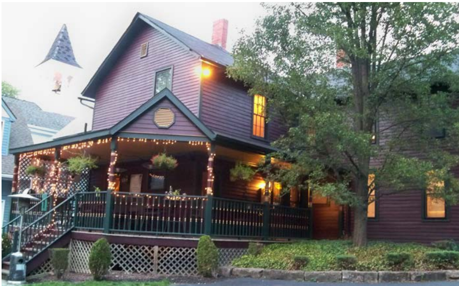
Williams put the back porch on the building.
