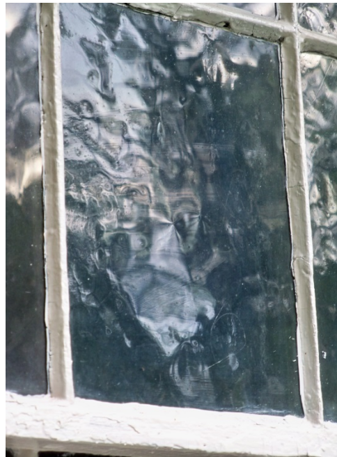
Some of window panes have been in the house since the 1800s. The surface is not as smooth as modern glass.
