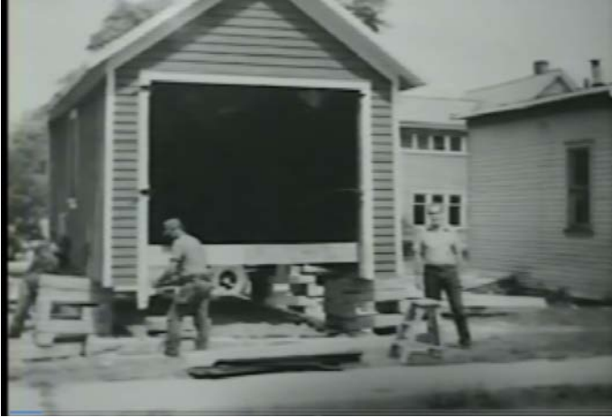
Like most Grand Pacific Junction buildings, the jail received a new foundation made of sandstone. Photo courtesy of Clint Williams.
