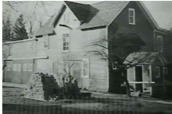
Here is the Livery Stable during the process of renovation and creation of Grand Pacific Junction. Note that the outhouse is farther from it. Photo courtesy of Clint Williams.
