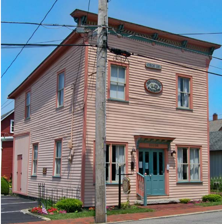
The Warehouse, which houses A Time to Spa, now looks like this, but it was in bad shape when Clint Williams acquired it in 1989.
