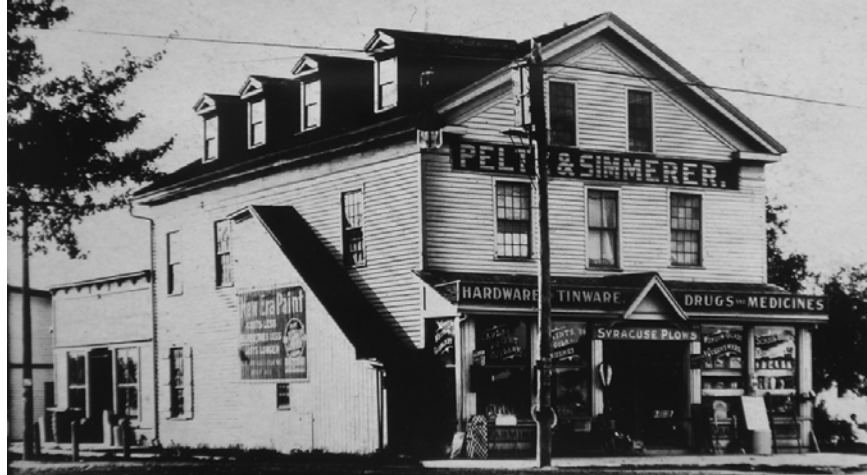
The enclosed stairway on the side of the building provided access to the medical and dental offices on the second floor. Clint Williams removed it when he remodeled the building while developing Grand Pacific Junction in the early 1990s.
