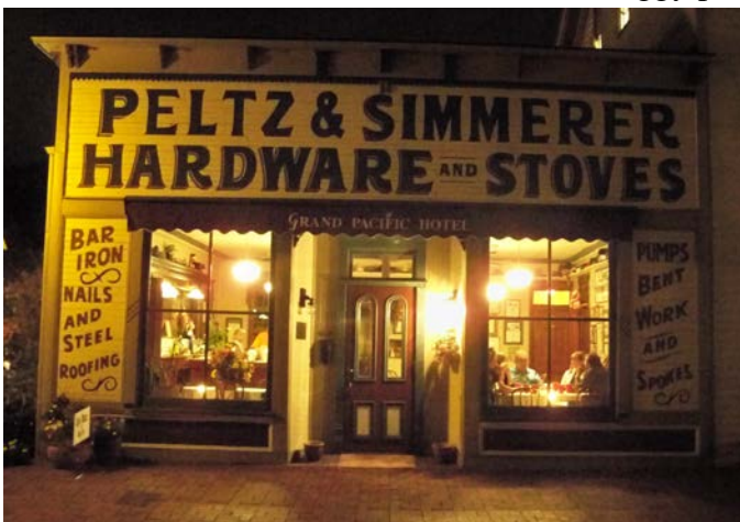
The side of the Grand Pacific Hotel reflects its former use as a hardware store.
