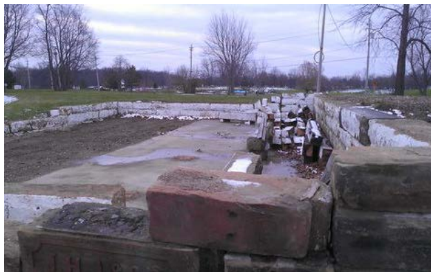
This was all that was left at the site on November 29. Photo by Bob Buzzard.
