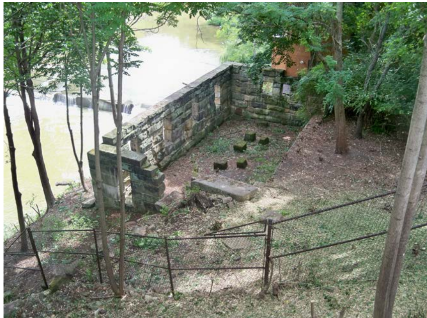
The view of the Damp's Mill foundation is now clear. The wall, which stands 13 feet tall, once supported a two-story wooden structure.
