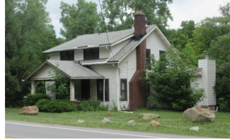
Before they moved to the big house up the hill, Theodore Herman TeGrotenhuis, his wife Mabel and their family lived in this house by Minnie Creek. In the mid-1900s, it was the home of artist Eva Cox.
