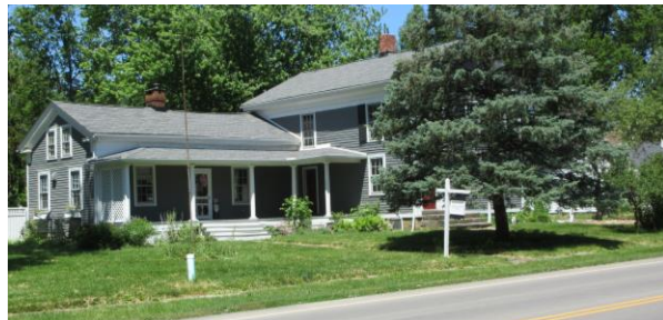
This house at 7622 Columbia Road is where Samuel A. Lay and his two wives lived in the late 19 th century.
