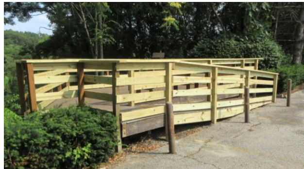
This new platform behind Falls Family Restaurant has replaced the old platform overlooking the foundation of Damp's Mill.
