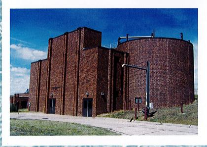
Anaerobic Digestion: Solids removed in the primary clarifiers are pumped to the primary anaerobic digester. Here the solids are decomposed in the absence of oxygen. The optimum temperature for digestion is 95° F. These solids are then transferred to the secondary digester where they are allowed to undergo further decomposition. During the decomposing process, methane gas is produced. This gas is stored in the secondary digester.
