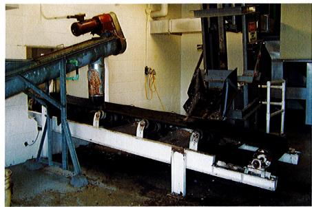
Screening: Before wastewater enters the wet well in the influent pump station, it passes through a mechanically cleaned bar screen which removes rags, sticks and other debris that may interfere with other plant equipment. A manually cleaned bar screen is provided in case the mechanical screen fails. The debris is conveyed to a trash dumpster in the loadout area.
