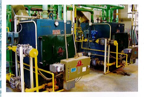
Methane gas produced in the anaerobic digesters can be used as an alternative fuel source. At this facility, it can be burned in either of the heating boilers. The boilers are used for heating the on-site buildings, as well as the sludge. The facility is designed to utilize a minimum of 95 percent of the methane gas produced.
