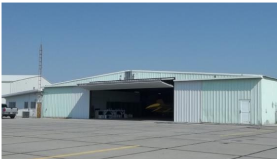
Storage Hangar with office on left (Bldg 3)
