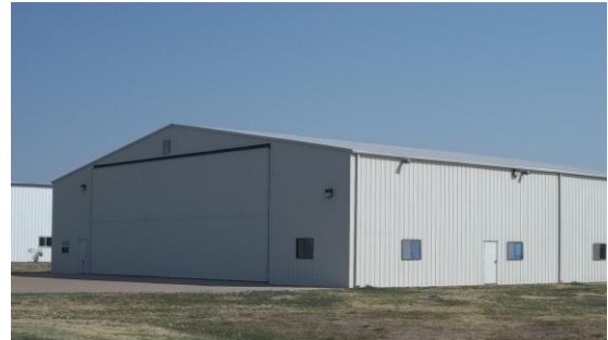
Storage Hangar (Adams Bank) (Bldg 2)
