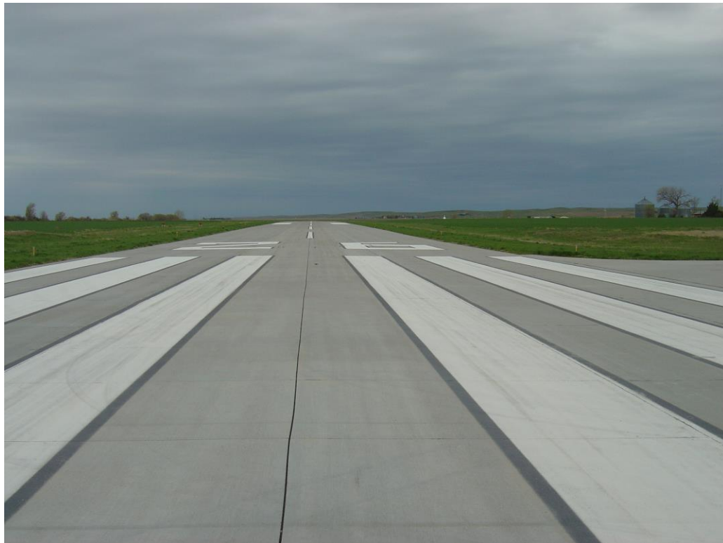
(Runway 26 looking west)
