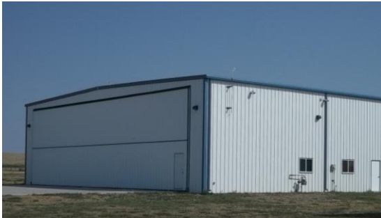
Hangar Leased by State Patrol (Bldg 1)
