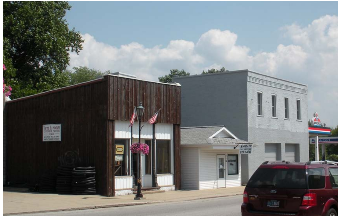
Typical commercial, retail and office in Town Center Middlebury.
