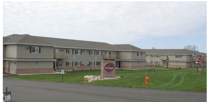
Heritage Estates Apartments
