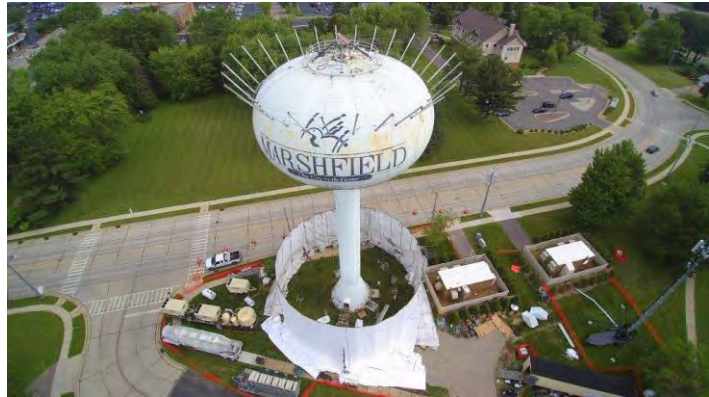
West Doege Street Water Tower being painted in 2016
