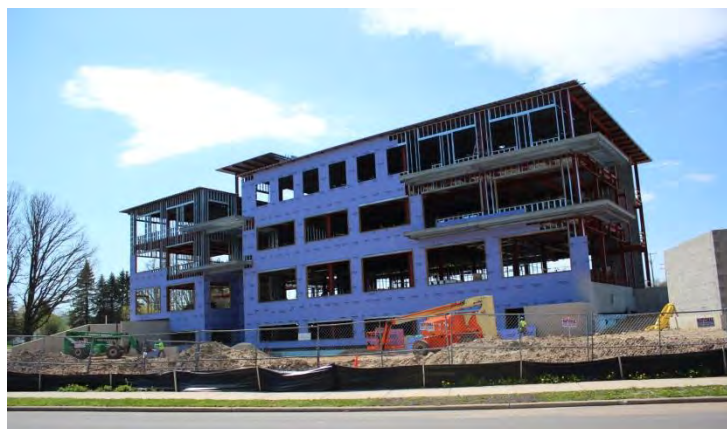
Construction of Forward Financial Bank Headquarters in TID #9 (2017)
