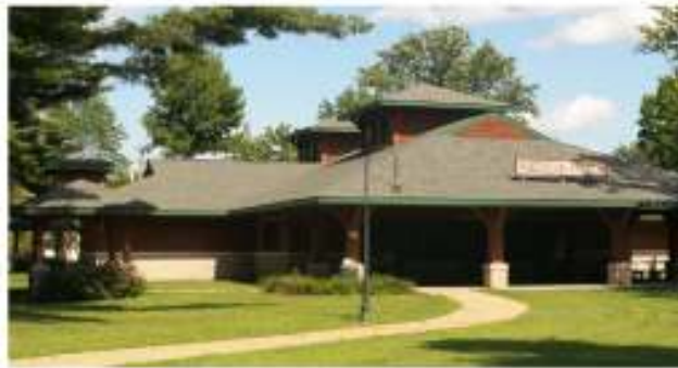
420-2749 Wildwood Station Building Rain Gutters
