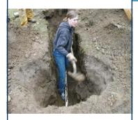
Challis digging a trench to repair a water leak
