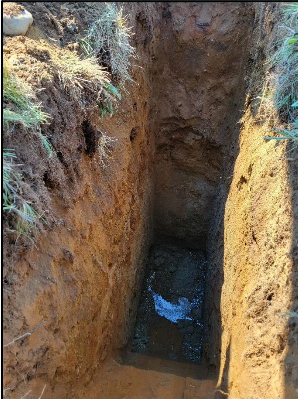
Image 2. Photo of TP-2 displaying granular soils and the observed perched water at 8.6' BGS. Image taken on 6.22.23
