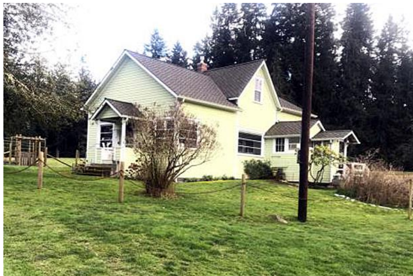
2017. Exterior restoration complete.
